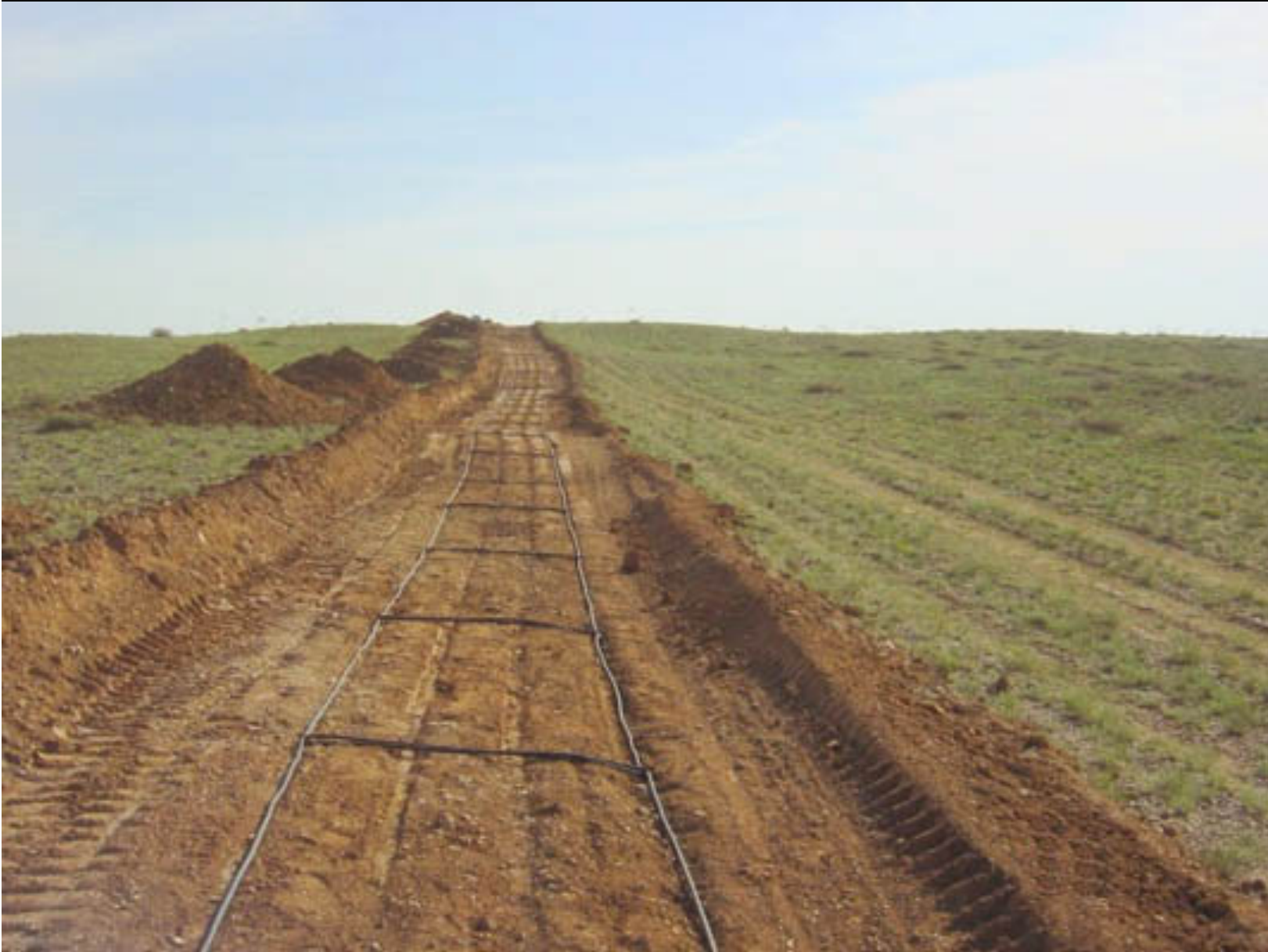
G-Max UPDS Perimeter Intrusion Detection system
